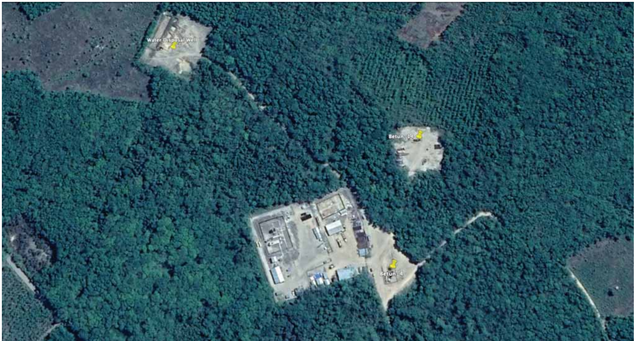
Gathering Station & Well Site
